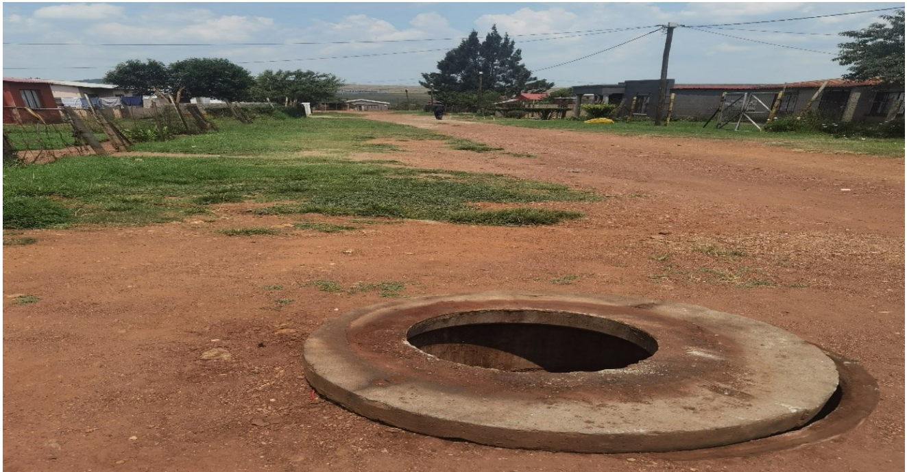
An exposed manhole at Nkanini.
